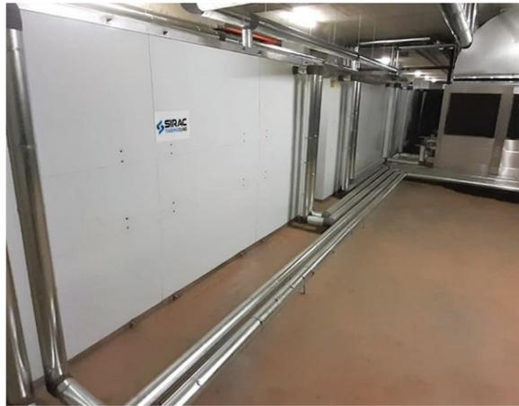
SIRAC supplied and installed: 3 x 17,500L **THERMOCUBE™** Tanks coupled with 6 x 90kW SIRAC Heat Pumps providing hot water for the Jewel City (Ithemba Properties) Development.
