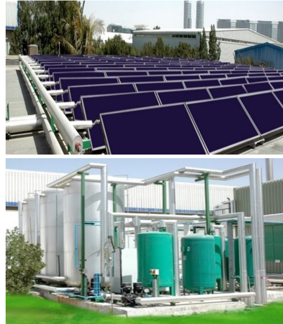
Forced circulation - Pumped
