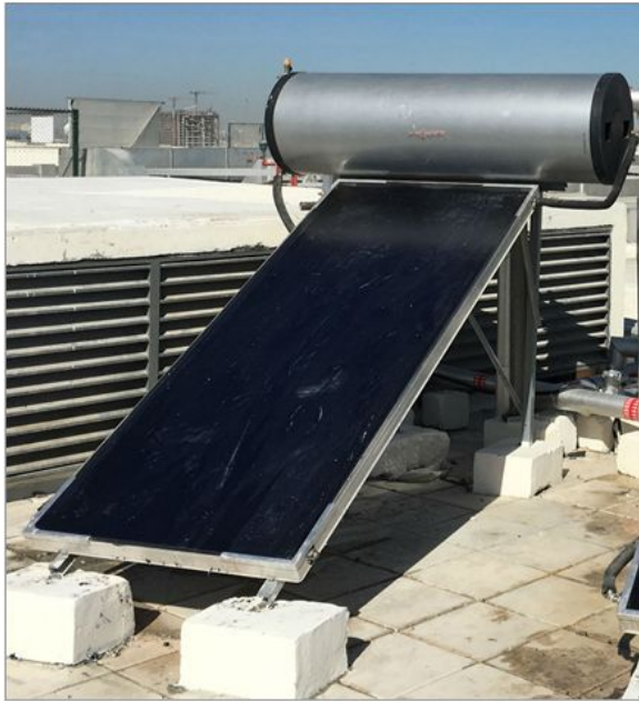
Thermosiphon - Gravity fed
